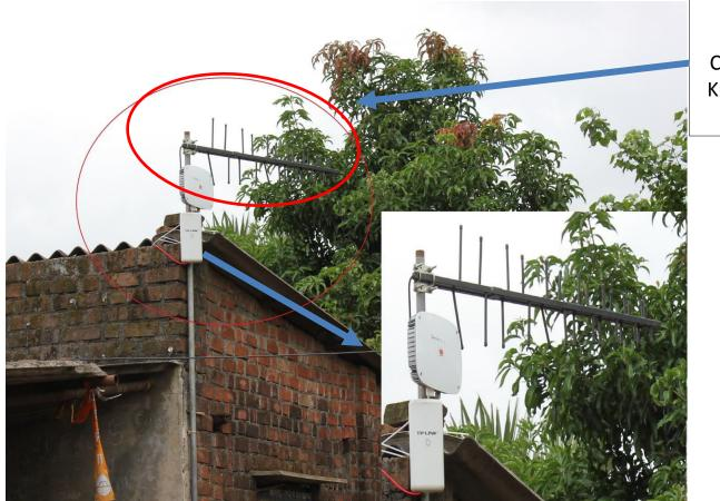
UHF Band Antenna Connected to Khamloli Base Station
