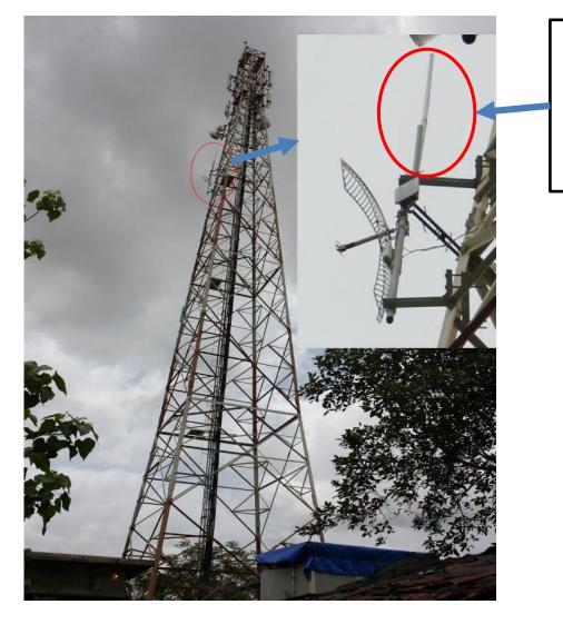
UHF Band Omni Antenna (500-520 MHz) Connecting Four GBTs
