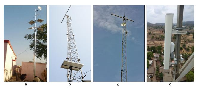
Fig. 3: The pictures show the devices installed at various villages in Unlicensed Band testbed. a) PBE-5AC-500 installed at Kev along with 48 V solar panels, b) PBE-5AC-500 installed at Shilshet along with 48 V solar panels, c) PBE-5AC-500 installed at Girnoli and d) LigoDLB 5-20 mounted on Maswan tower.
