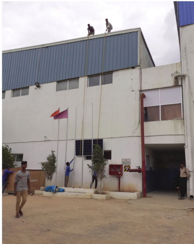
Figure C.2: Risky manual handling practice.
