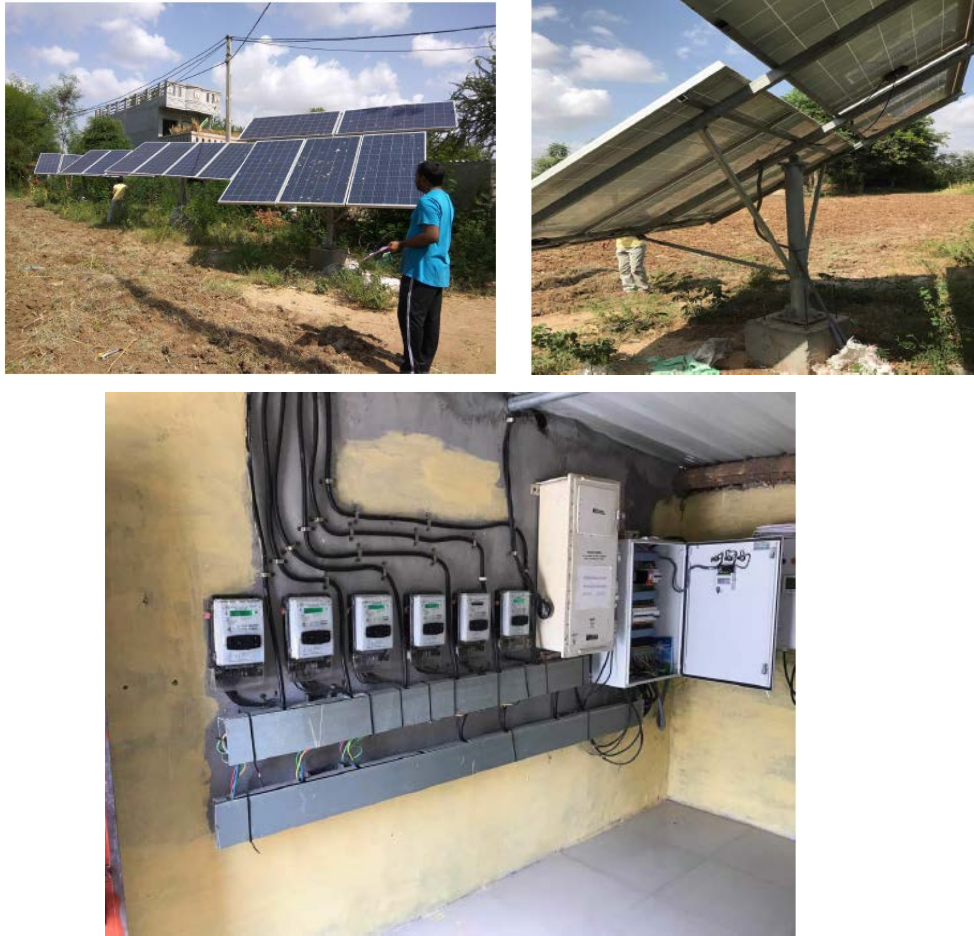
Figure 7.18: PV installation in the field and the meter room at Dhundi.
