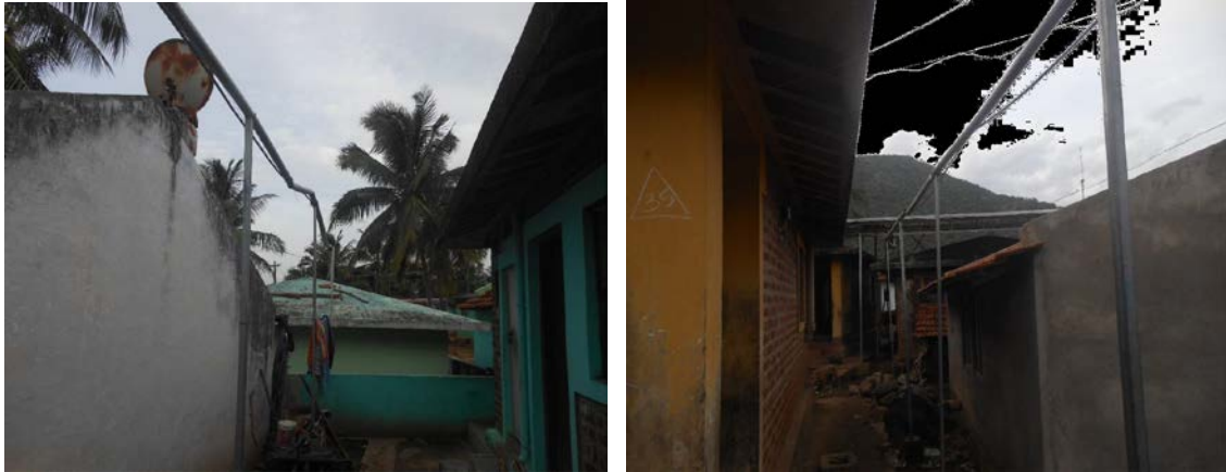
Figure 6.4: Power lines drawn through private spaces causing safety risks and hindering free movement of inhabitants.
