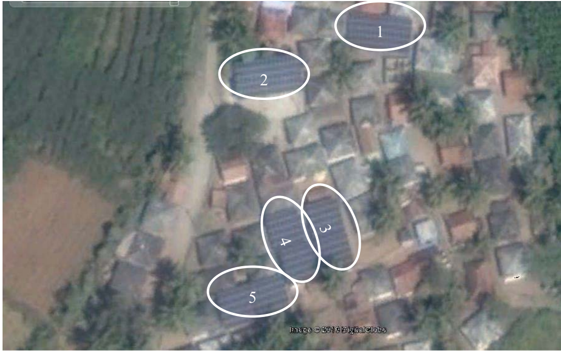
Figure 6.3: Satellite view of Chalayoor hamlet with the rooftop PV systems.
