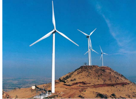
Four -1500 KW Wind Turbines installed in Davangere, Karnataka
