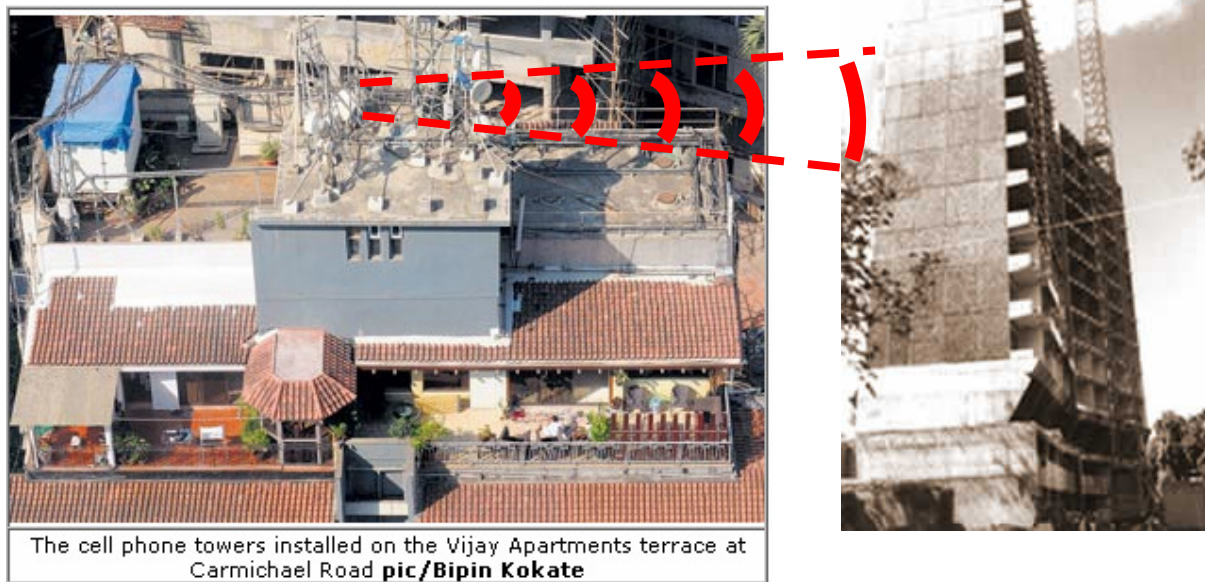
Fig. 2 – Cell phone towers installed at the roof top of a building in Mumbai
