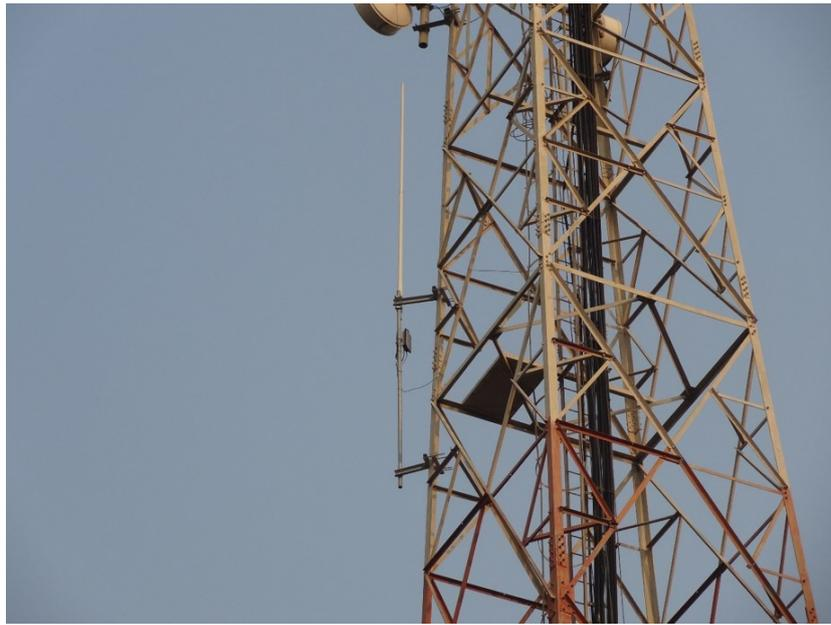
Figure 4.13: UHF TV band Access Point deployed at Khamloli tower
