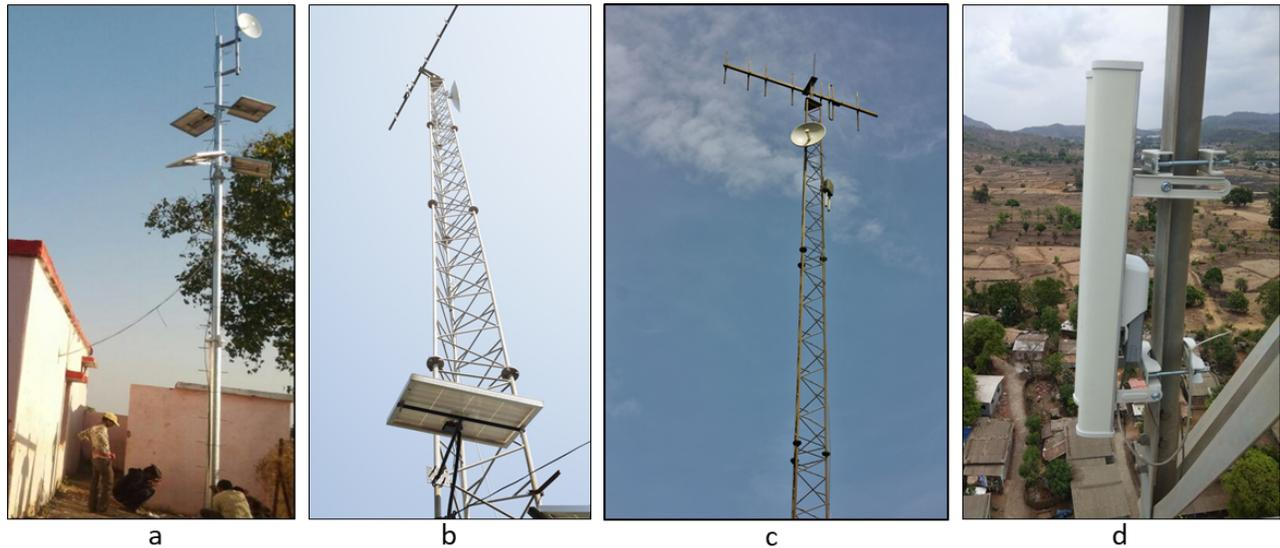
Fig. 3: The pictures show the devices installed at various villages in Unlicensed Band testbed. a) PBE-5AC-500 installed at Kev along with 48 V solar panels, b) PBE-5AC-500 installed at Shilshet along with 48 V solar panels, c) PBE-5AC-500 installed at Girnoli and d) LigoDLB 5-20 mounted on Maswan tower.
